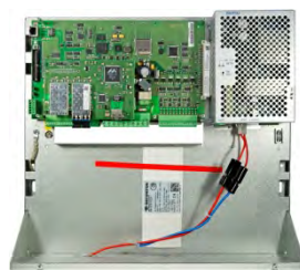
Fig. 57 Main processor unit and power supply unit
